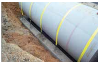
Washing of underground tanks
