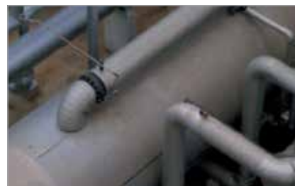
Washing of refinery systems
